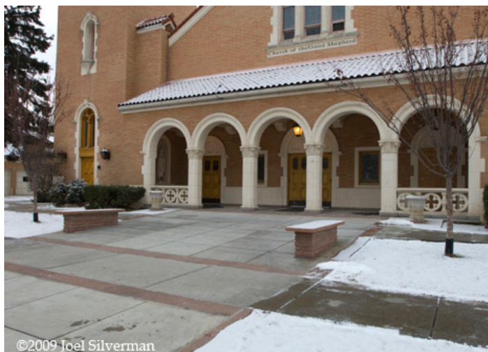
This photo is of a church in Vail, Colorado. They use Easy Heat snow melting mats embedded in the sidewalks. (Courtesy of Easy Heat.)
