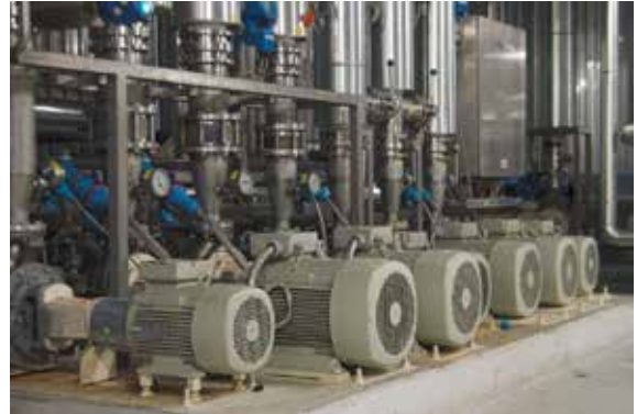
Monitor electric motors for leakage to earth in a pump station.
