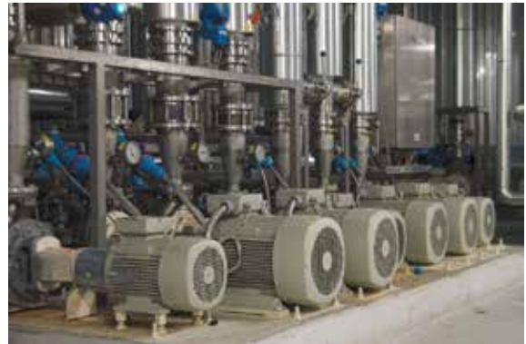
Monitor electric motors for leakage to earth in a pump station.
