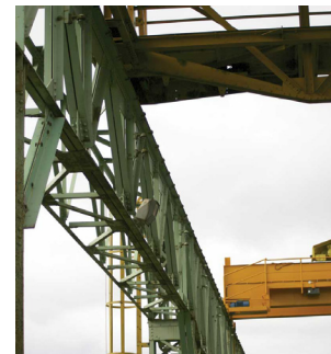
Gantry Cranes often use DC powered motors for high torque at low speed.
